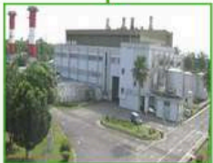
TUNKU ABDUL RAHMAN (BIAWAK) POWER STATION (66 MW)
