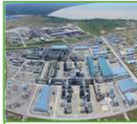
BINTULU GAS POWER PLANT (1,140 MW)
