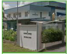
MIRI POWER STATION (50 MW)
